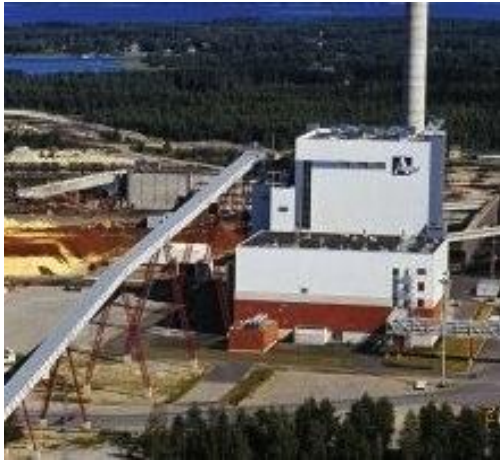
Alholmens 240MW – World's largest multifuel boiler
