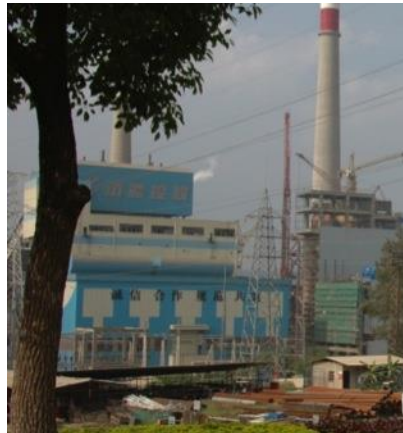
Sha Lang Tan 300MW – China's largest FBB
